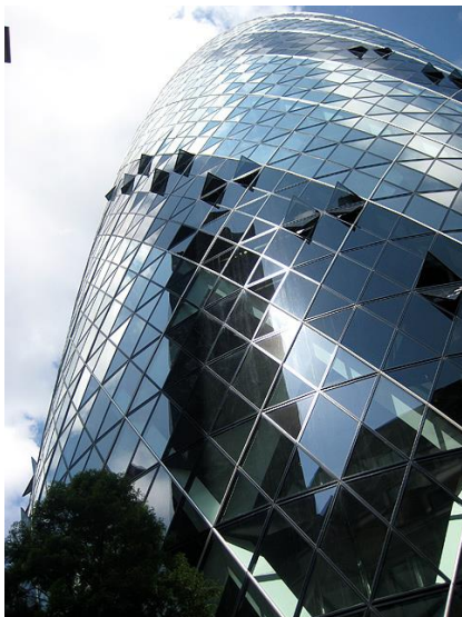
30 St Mary Axe – showing triangular openings in the outer skin
