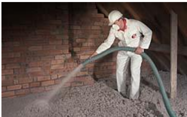
Dry loose-fill installation
