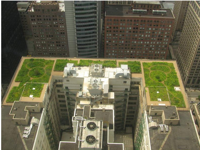
Green roof on Chicago City Hall, November 2008
