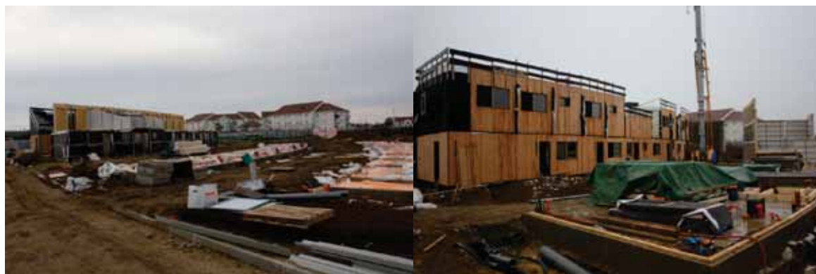
Photograph 1 and 2: the building site in November 2009 et February 2010
