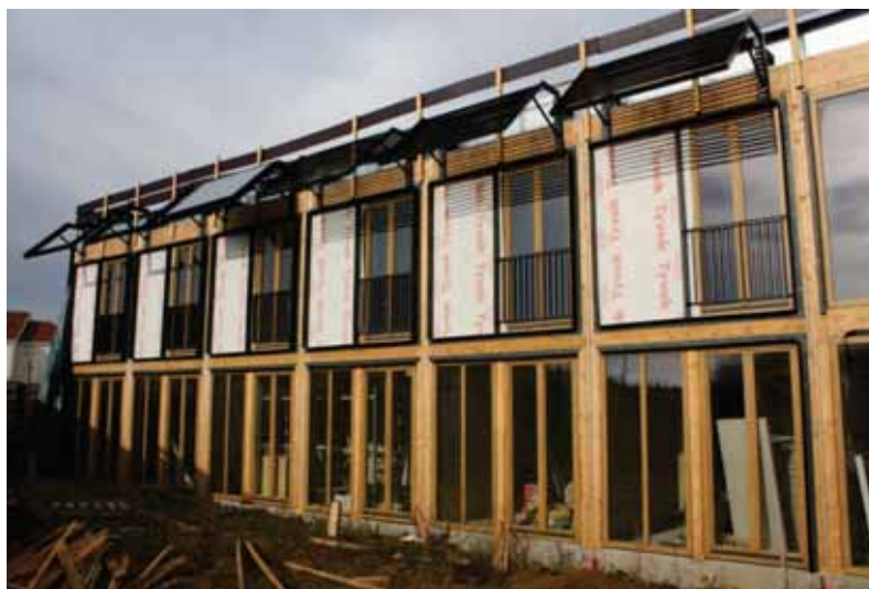
Photograph 5: Structures that will support solar panels and prefabricated façades
