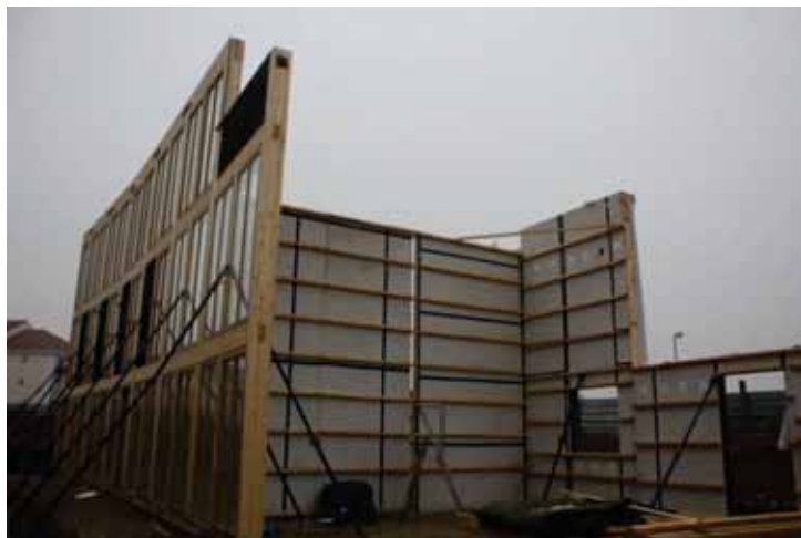
Photograph 3 : façades (9 meters) prefabricated in Serbia
